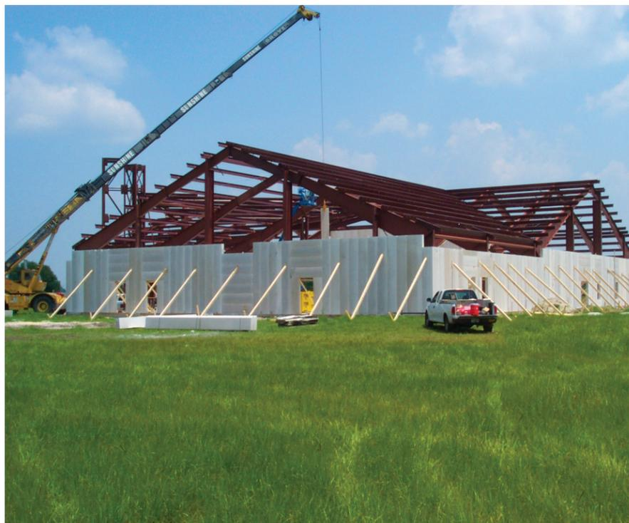
Panels made of Hebel® AAC form 4-, 8- and 12-room pods. These permanent yet flexible structures are ideal replacements for temporary classrooms. They can match existing campus architecture or be used for complete campus construction. On a proper foundation, additional floors can even be added for increased square footage.
